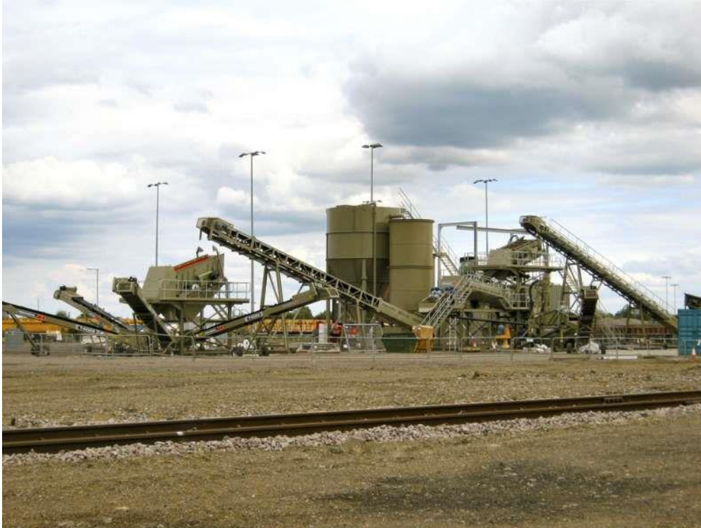
Figure 5: Ballast treatment facility 32
